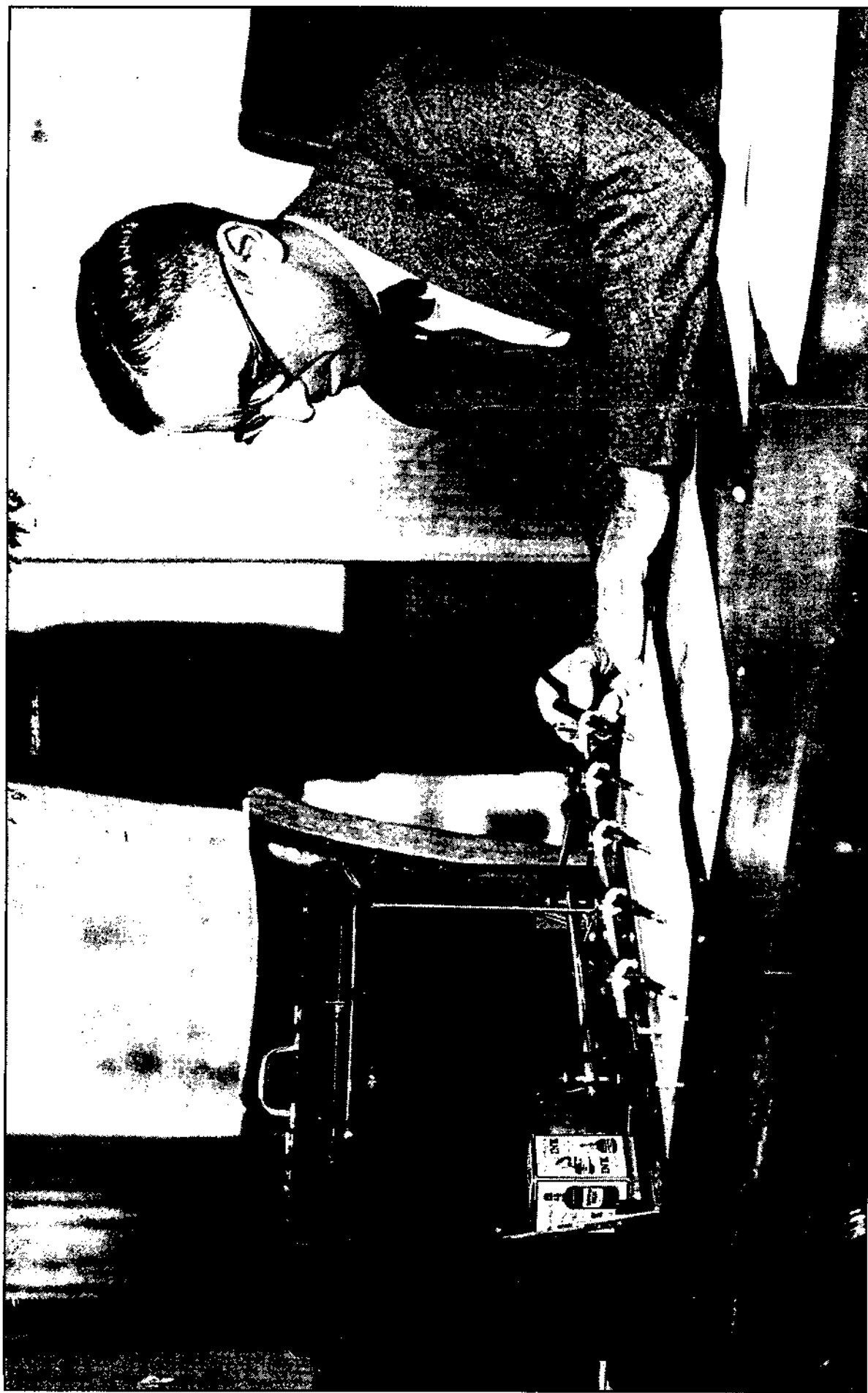
Figure 5. This shows that Truman did like to use a pantograph with a master and five slave pens.
